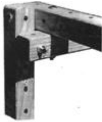
Figure 9. Bolting of three pre-drilled members for a solid connection.
