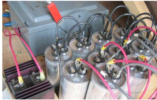
Figure 19. Capacitors used in initial testing of the electric motor.
