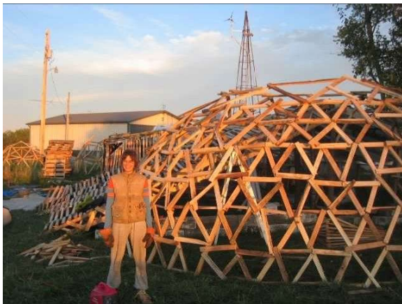
Figure 4. Living dome under construction.
