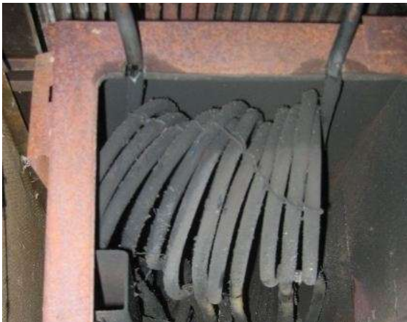
Figure 31. Heat exchanger coil inside a stove for warming up the lettuce bed.
