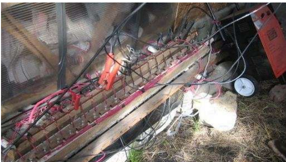
Figure 9. Twelve volt battery bank with reserve capacity of approximately 900 amp hours (~9 kWhr). Standard 40 amp automotive battery charger is in the back. The long structure above the batteries is a homemade voltage switcher from 12 to 120 volts DC.
