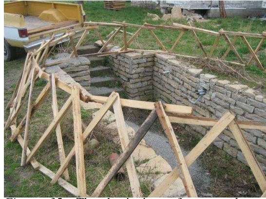
Figure 35. The beginning of sprout house construction.
