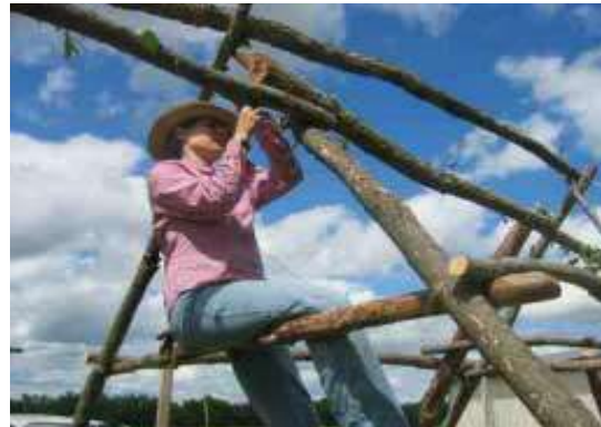
Figure 2. Greenhouse under construction.
