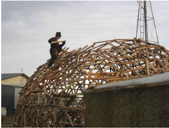
Figure 3. Workshop under construction.
